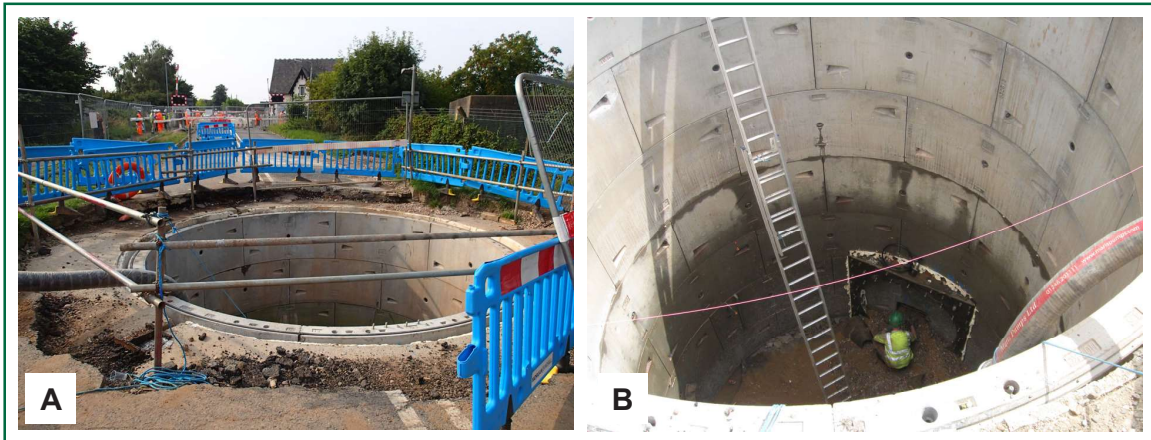
Figure 6: Launch shaft (a) and reception shaft (b) during the works (image courtesy of Morgan Sindall)
